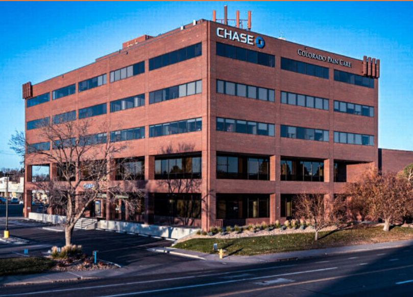
2696 S COLORADO BLVD (WEST)
